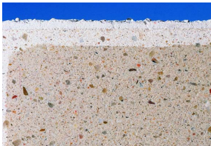
Figure 4: Penetration of a primer into limestone
